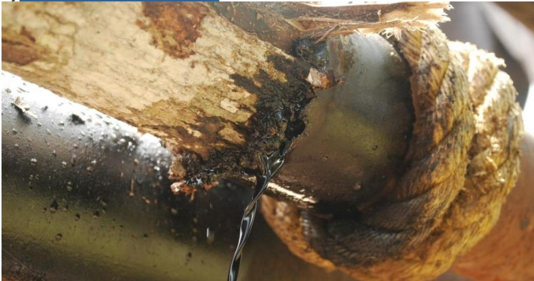
A close-up of a leaking pipeline, stuffed with a tree to stem the oil flow. (Photo: [newmy51/cc/flickr](#))
